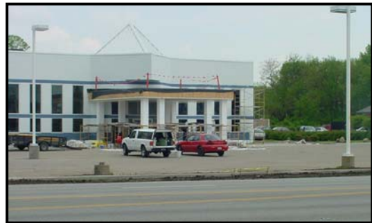
Substantial Renovation – Northern Section of Route 4
