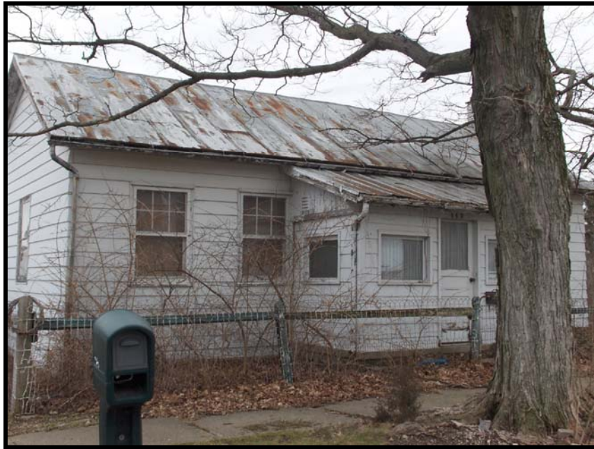
Roof in need of repair, rotting fencing 142 Jefferson Street
